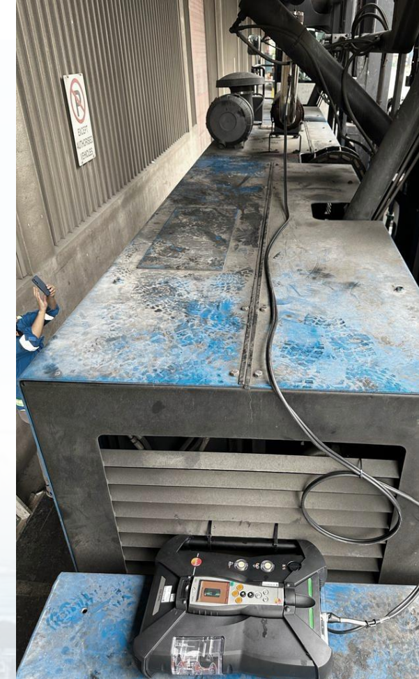
Gas analyzer control unit set secured on the back of the side loader
