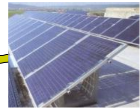
Airport T3 system
