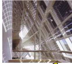
BCA PV system
