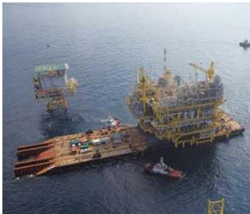
Floatover Installation for offshore platform (Courtesy: McDermott)
